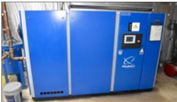
QUINCY 50-HP QCV-50 ROTARY SCREW AIR COMPRESSOR
